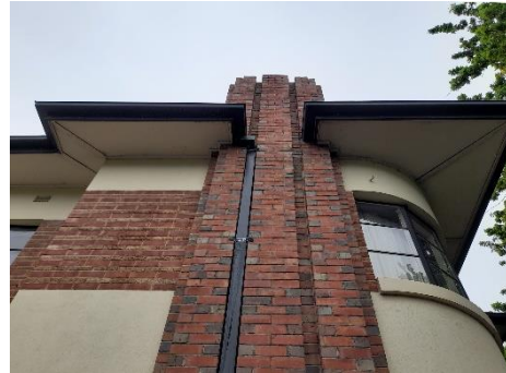
Tower containing chimney
