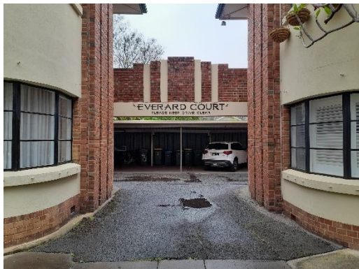
Driveway between blocks with beam over
