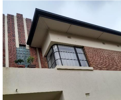
Upstairs window showing curved glass
