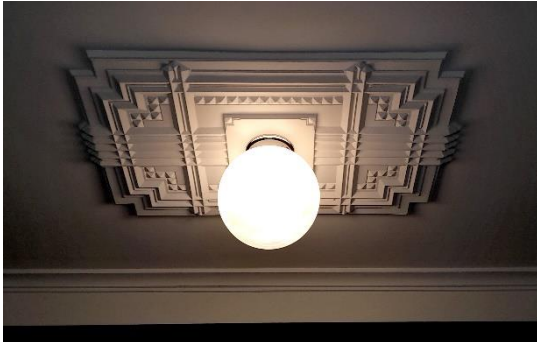
Typical ceiling rose
