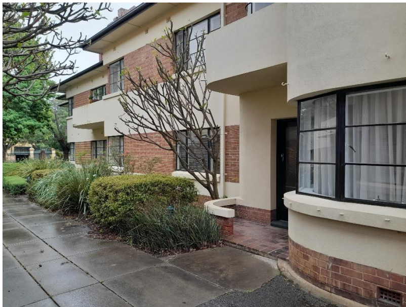
East Wing, view towards Anzac Highway
