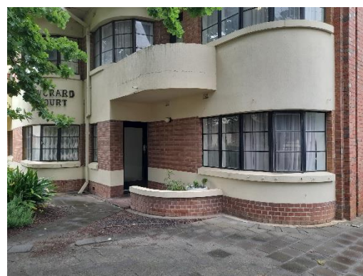
West wing showing cantilevered balcony and porch dwarf wall
