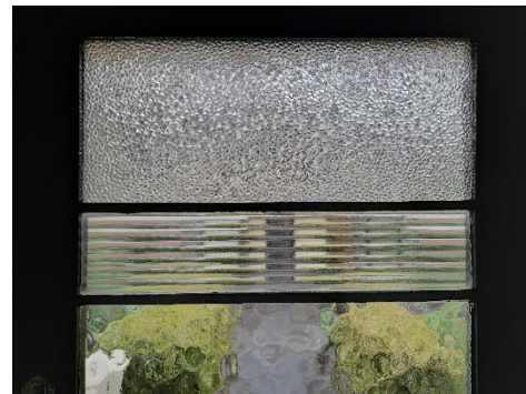
Doors to common stairwell showing chromed muntins, reeded and patterned glass
