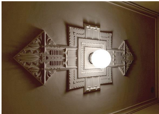
Typical ceiling rose
