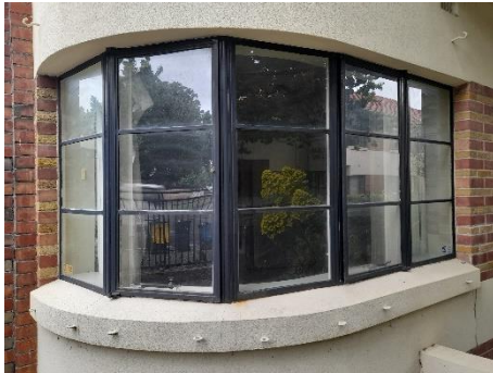
Segmental steel casement window frame
