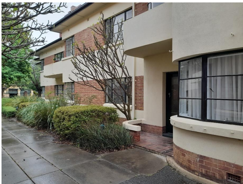
East Wing, view towards Anzac Highway
