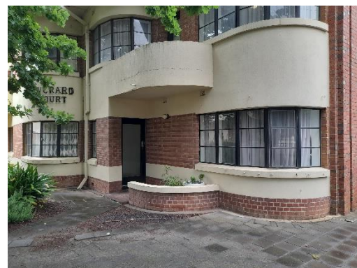
West wing showing cantilevered balcony and porch dwarf wall
