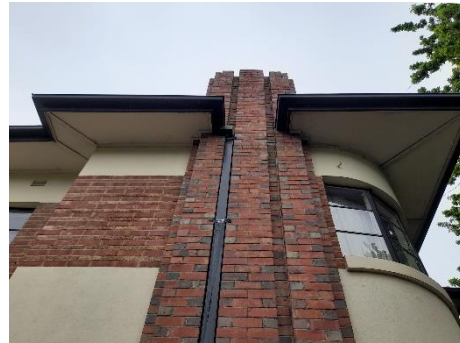
Tower containing chimney
