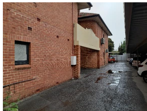
Rear view with carparking space on right
