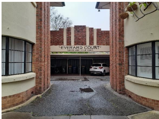
Driveway between blocks with beam over
