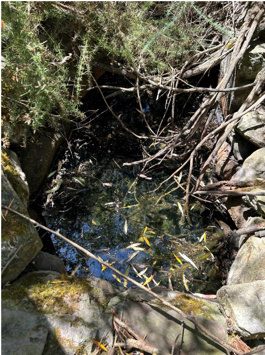
The stone-lined well at Sandergrove Water Reserve in December 2023.
