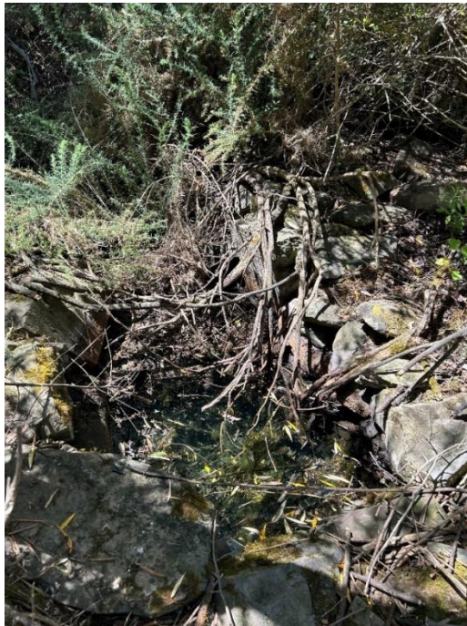
Stone-lined well at Sandergrove Water Reserve.
