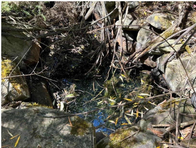
Stone lining to well created from a natural spring.
