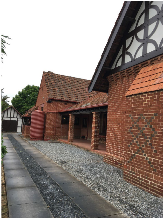
Western elevation looking north, showing garage and verandah accessed from billiard room and over which the dining room and kitchen have views. Note the curved imitation half-timbered bracing, and stepped and patterned brickwork to chimney.
