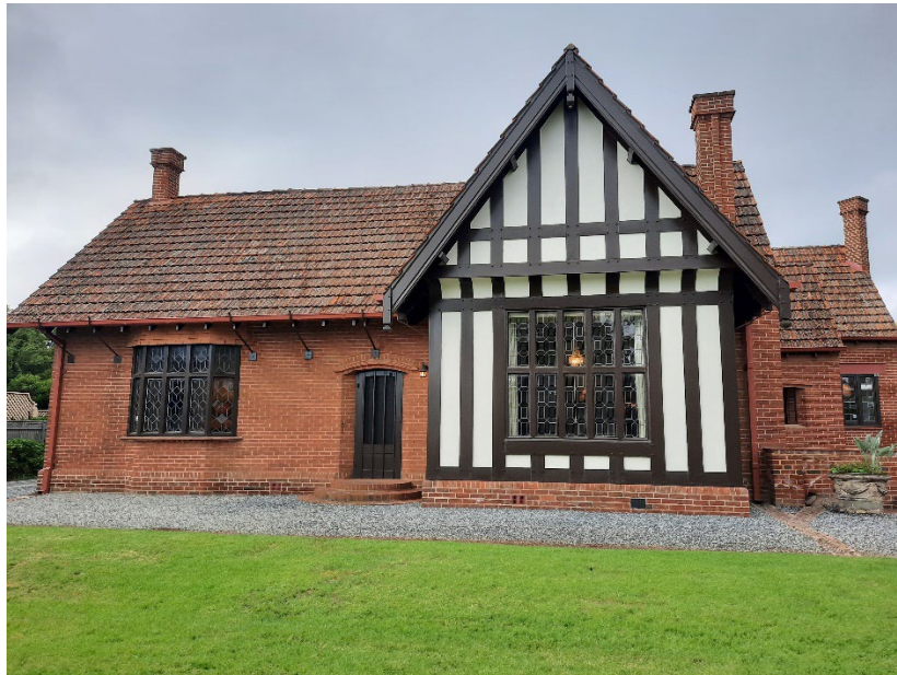
Southern elevation (facing Fitzroy Terrace), note domestic-scale, covered soffit between jettied gable and wall, imitation half-timbering, chimneys, eave brackets, and terra cotta roof tiles.
