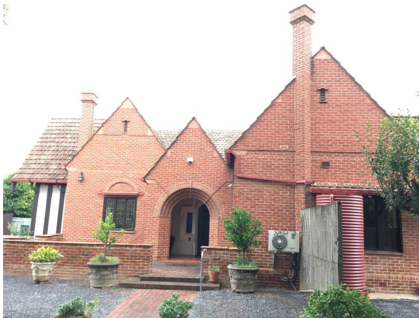
Part east elevation showing main entrance, note patio/terrace with stepped-brick detailing to arch, triple gables with Roman brick detailing, and arch feature over window.
