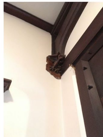
Detail, example of a gargoyle and timberwork in hallway.
