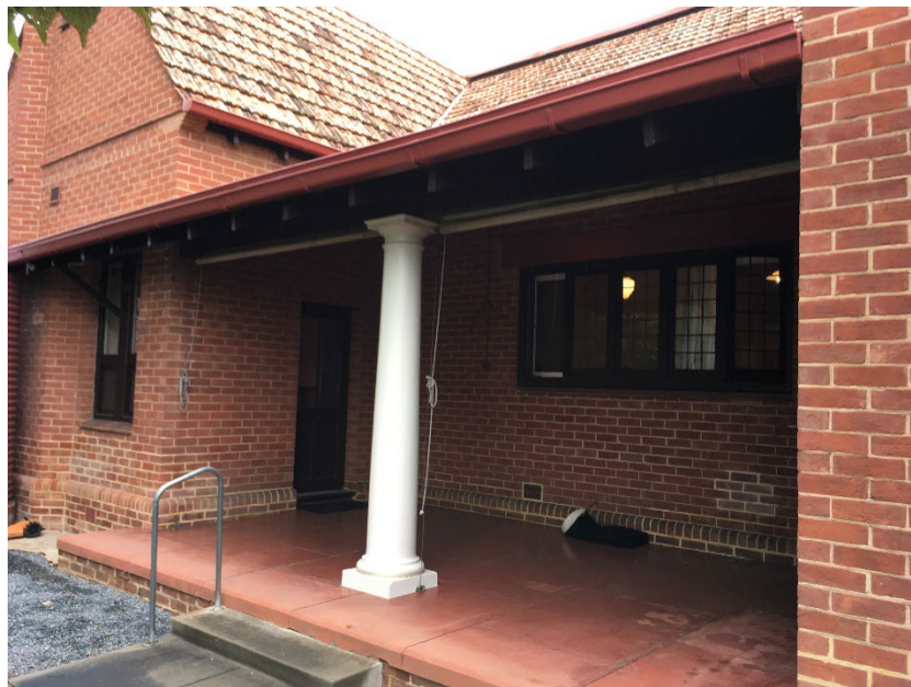
Part western elevation showing the verandah between master bedroom and second bedroom. Both bedrooms have access to the verandah, while the dressing room overlooks it. Note column, and red-brick plinth with curved red-brick capping.
