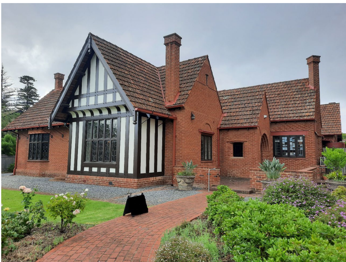
5 Fitzroy Terrace, south and east elevations
