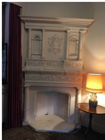
Detail, bespoke designed fireplace for the hall (painted concrete).
