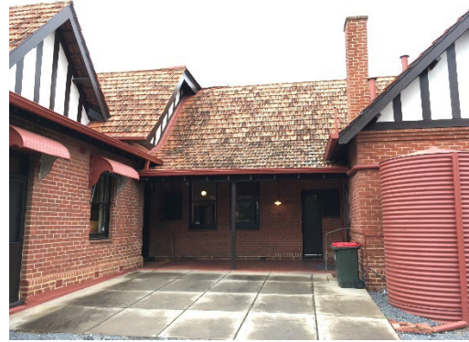
Views of the rear of the house, showing roof forms, verandah and imitation half-timbering to gables.
