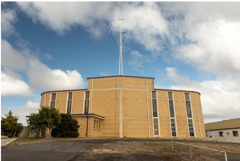
Rear view, showing sacristy block, clerestory section and spire
