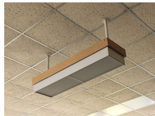
Flourescent light enclosure and suspended ceiling
