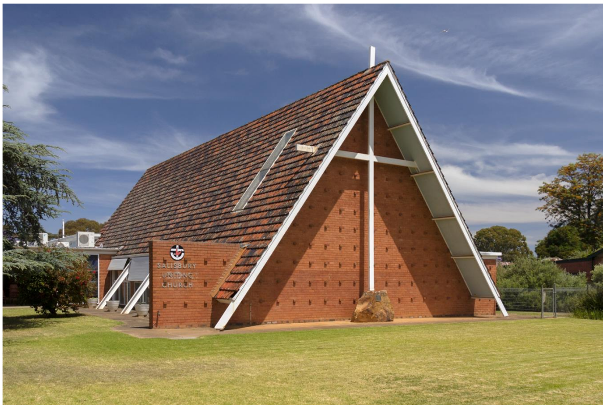
Former Salisbury Methodist Church, 2 November 2023
