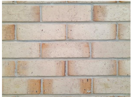
Face brick in chapel
