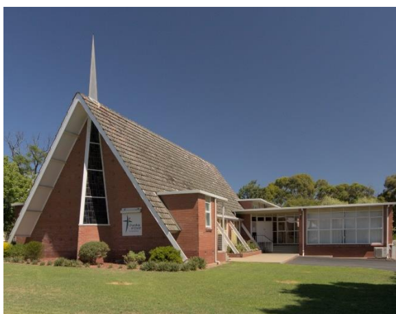
Naracoorte Church of Christ, 1966, is an example of a true A-frame church
