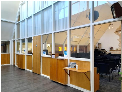
Glazed partition wall between foyer and chapel
