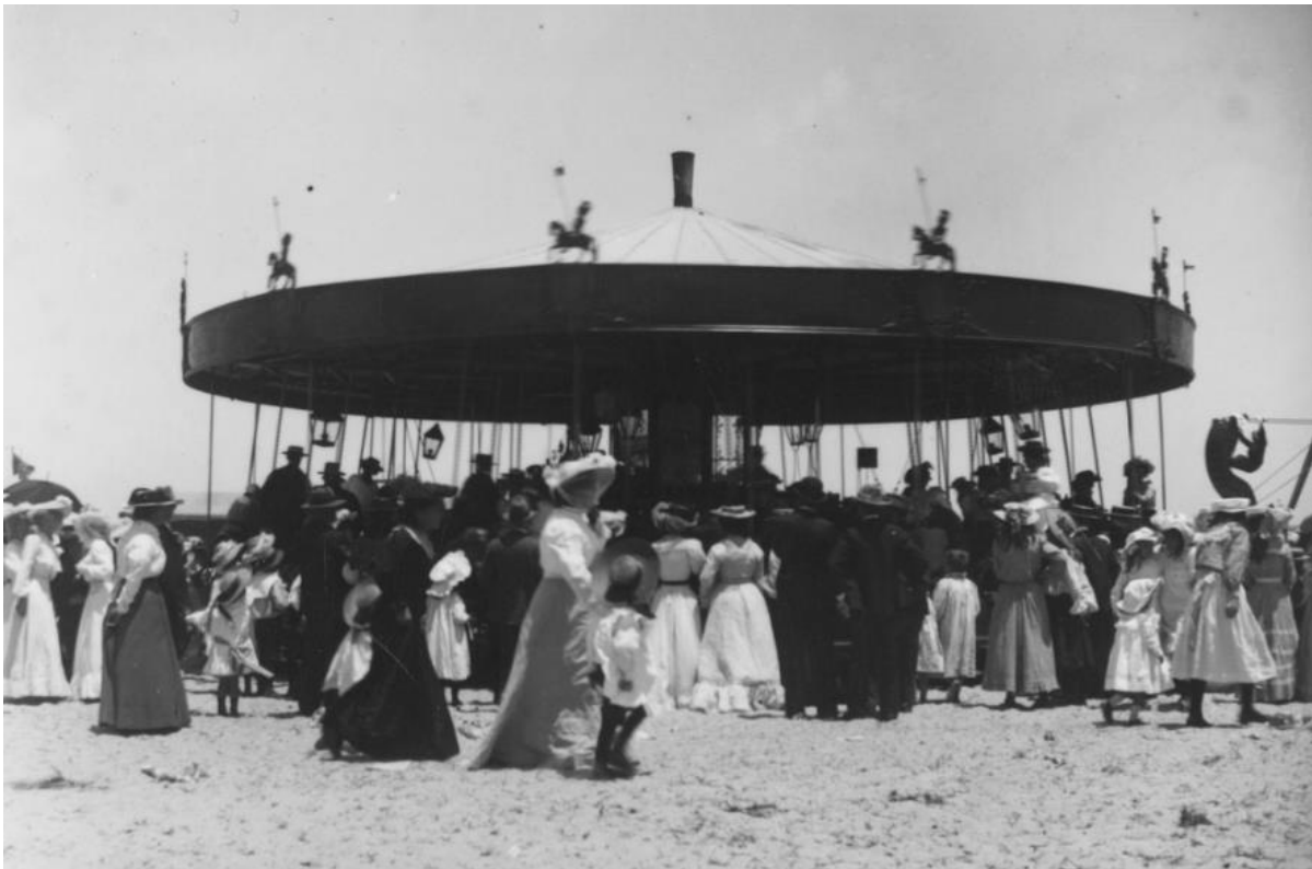
Believed to be E. A. Brown's steam-driven carousel, Glenelg, c1910, later sold to Pastimes Ltd and known as Pastimes' Royal British Riding Gallery, note central flue.
