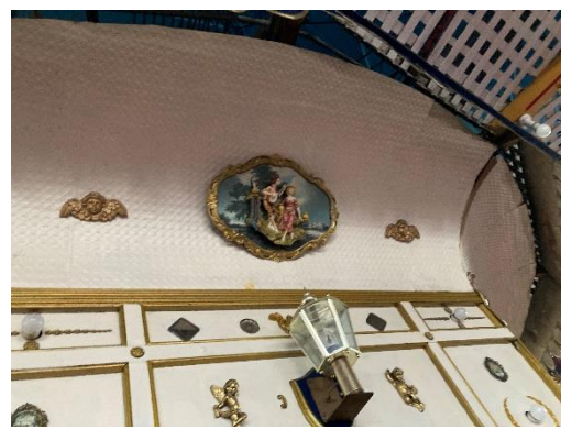
Pressed metal soffit to centre console, with applied decoration [not original fabric].
