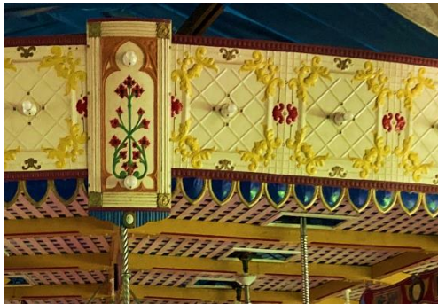
Pressed metal rounding boards (detail).
