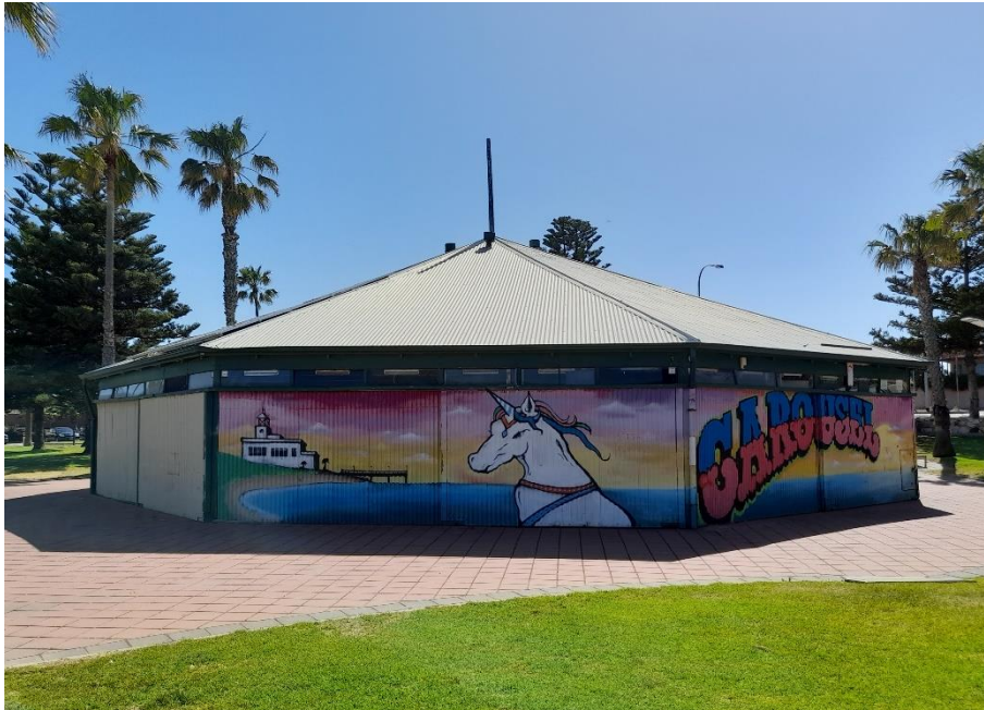
Semaphore Carousel Pavilion, showing clerestory windows, sliding doors (closed) and mast.
