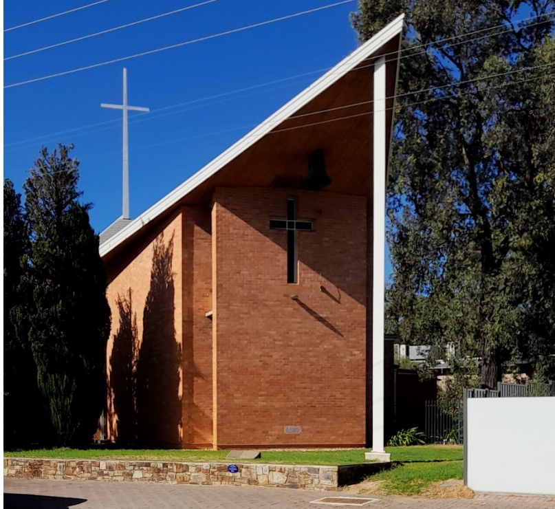
St David's Anglican Church, exterior from Glynburn Road
