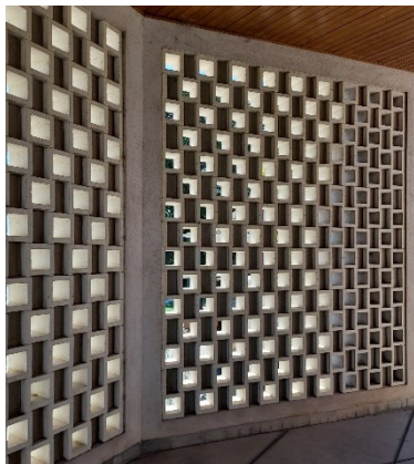
Porch blockwork screen
