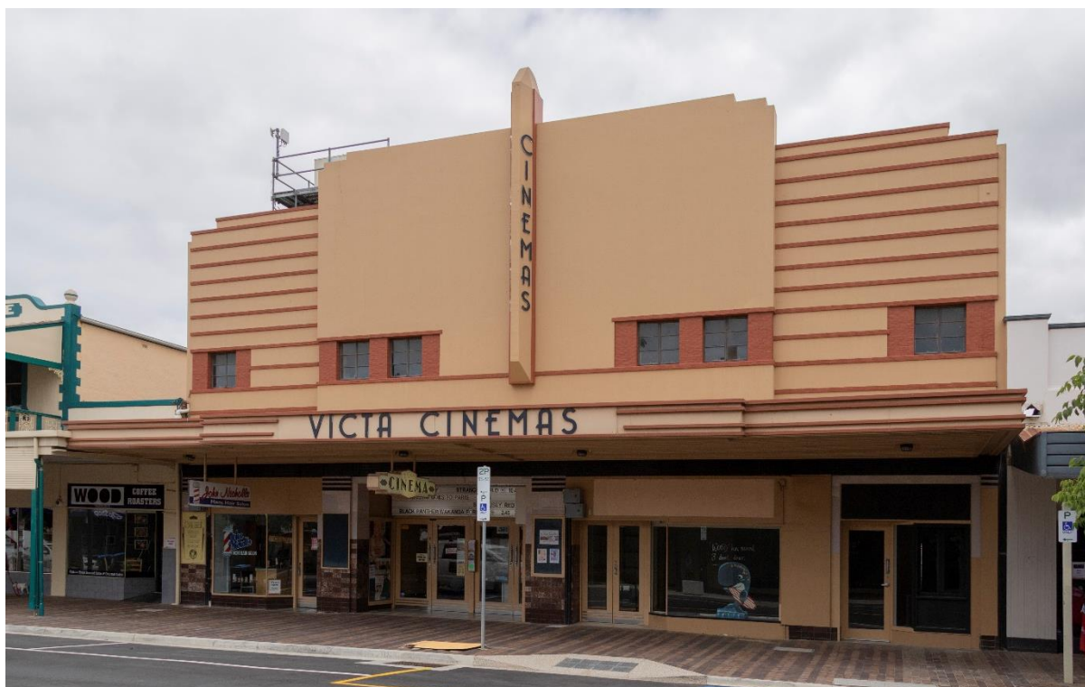
The Victa Cinema (former Ozone Theatre), 28 November 2022
