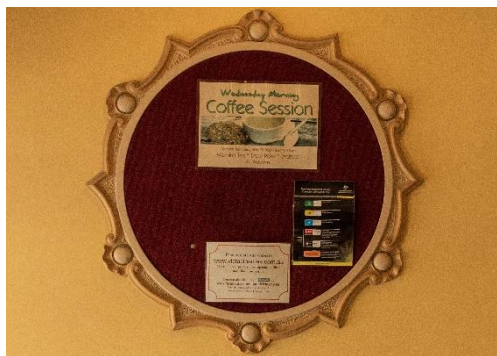
Notice board in vestibule, with fibrous plaster frame
