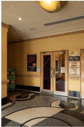
Vestibule showing terrazzo floor
