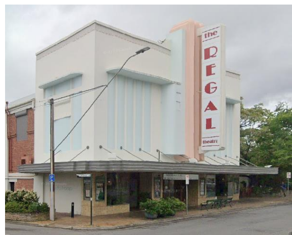
Chelsea Cinema, 275 Kensington Road, Kensington Park (SHP 10952)
