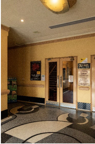
Vestibule showing terrazzo floor
