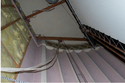
Original proscenium hidden behind screen with perforated fibrous plaster frieze at top
