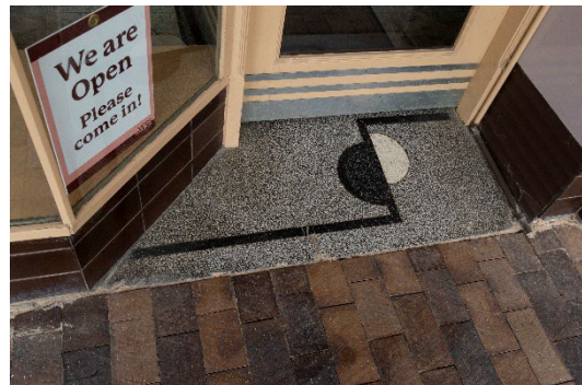
Terrazzo re-entrant floor to Shop 1
