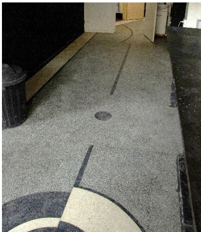
Side exit terrazzo floor
