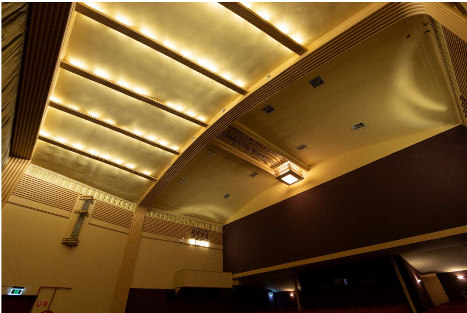
Downstairs auditorium ceiling
