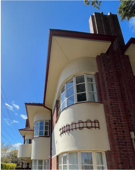
'Shandon' name plate and steel-framed casement windows.
