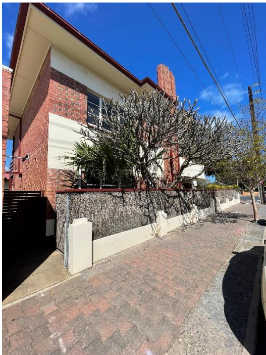
Northern elevation, with eastern elevation on left.
