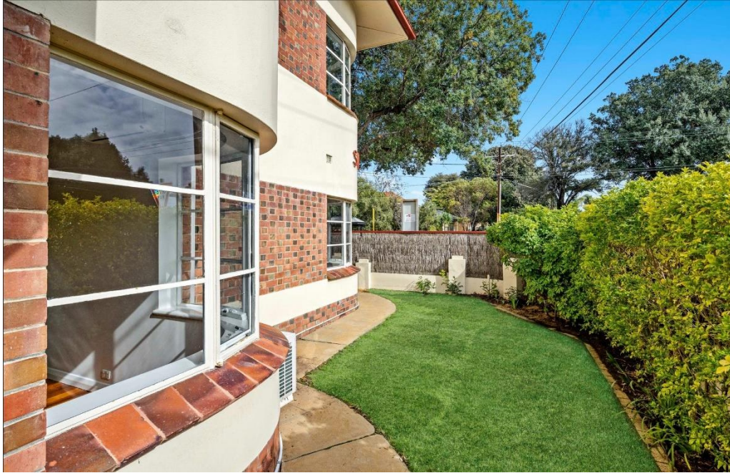
View of garden area looking westwards towards Moseley Street, showing steel-framed casement windows.
