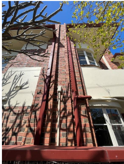
Northern elevation showing one of the chimney towers with Flemish bond coursework.
