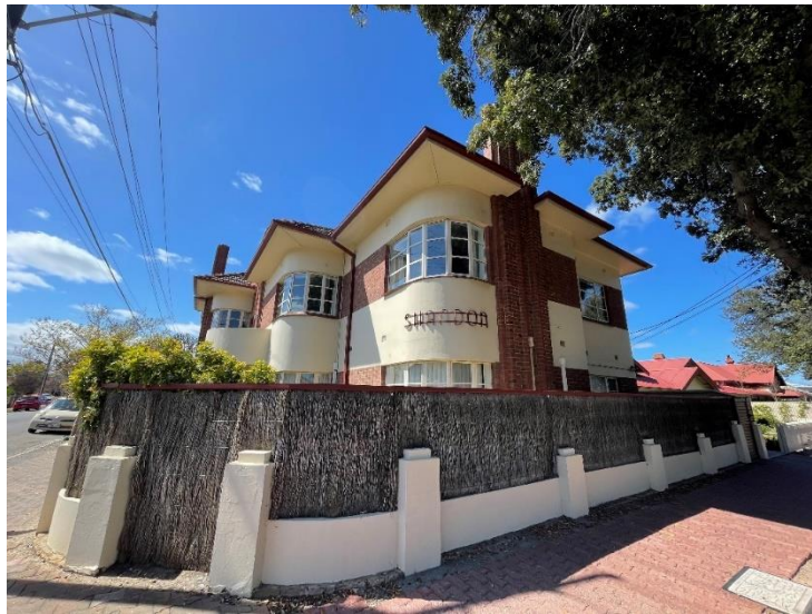
Shandon (flats) at the corner of Moseley Street and Bath Street, Glenelg South, note original masonry front fence.
