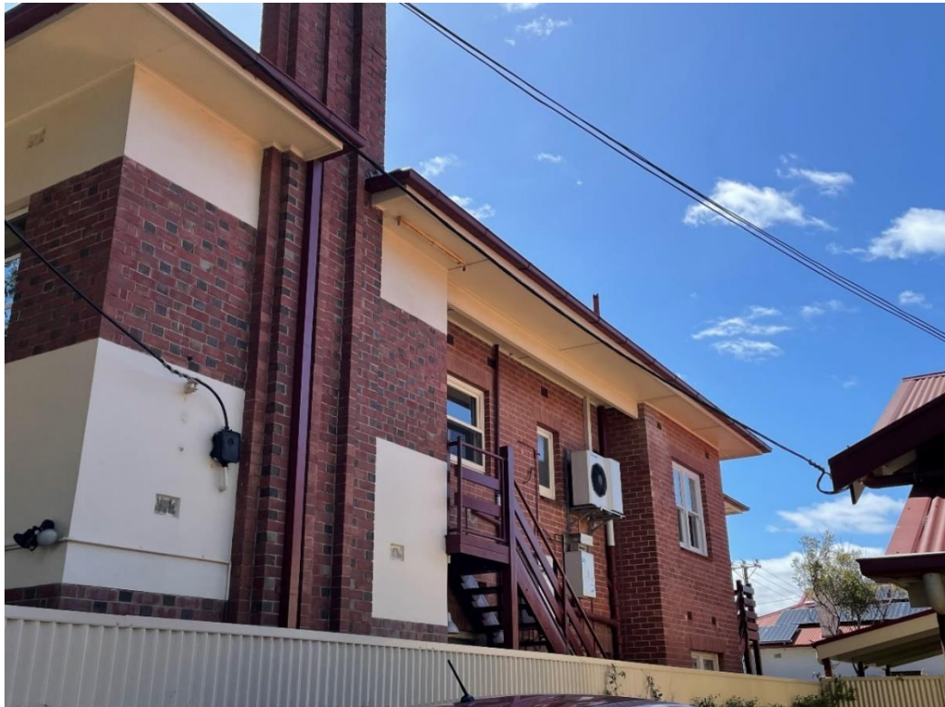
Southern elevation of Shandon (flats), showing timber staircases at rear.
