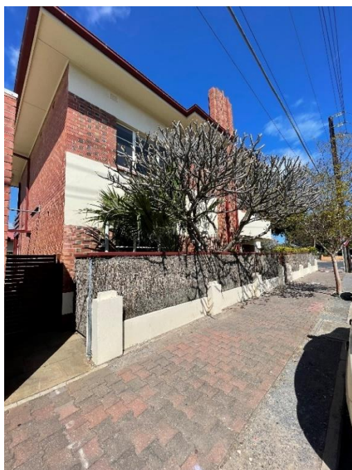
Northern elevation, with eastern elevation on left.
