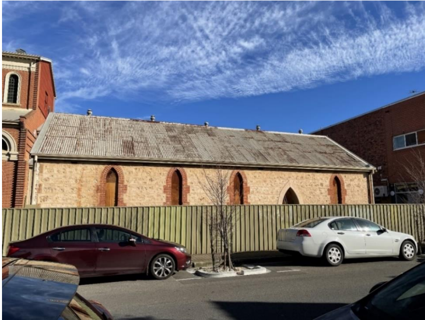
Eastern wall showing the original front entrance (on right) and windows with pointed arches and red-brick quoins.
