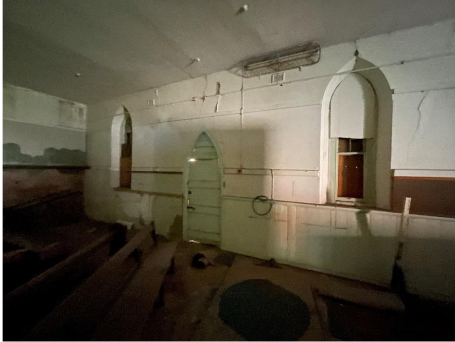
The interior side of the east-facing wall showing the original windows and entrance.
