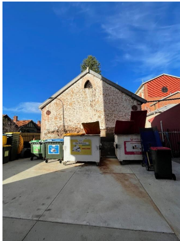
Northern wall of St Patrick's Schoolhouse.
