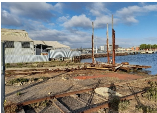
Large slip cradle in situ on site of former A. McFarlane & Sons Slip
