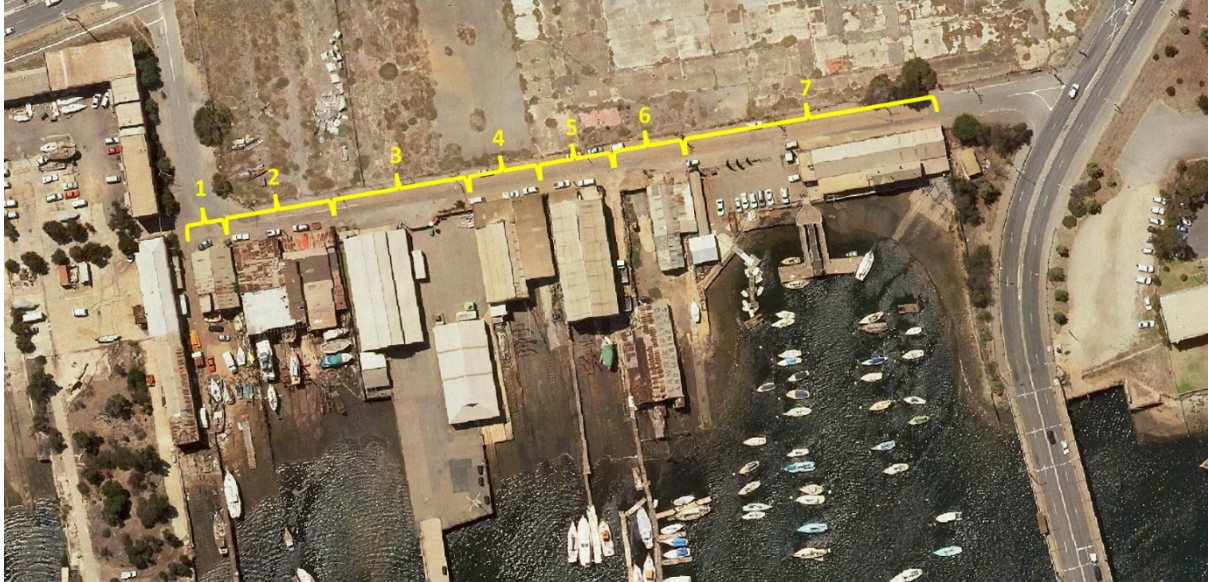
Jenkins Street Slips Precinct, aerial view, 2006, prior to removal of shipyard structures.
