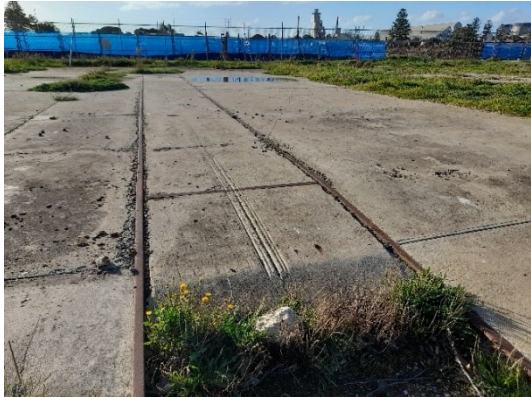
Detail of slipway showing floor slabs
