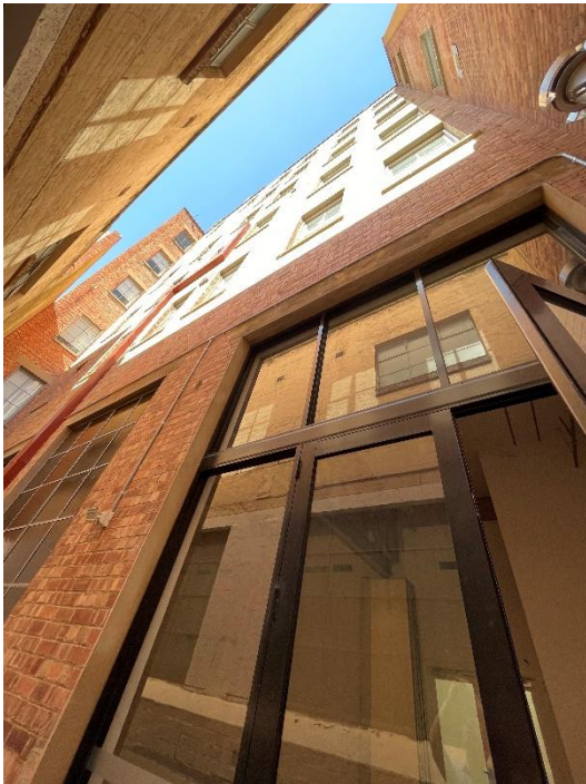
Retrofitted steel doorframe on the east.
