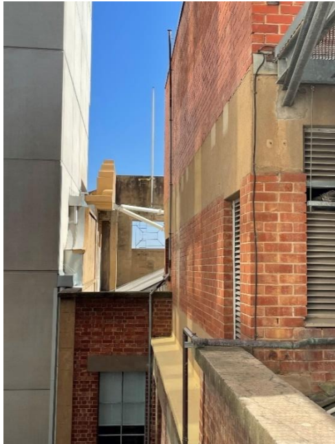
Partial view of the parapet wall from the rear.
