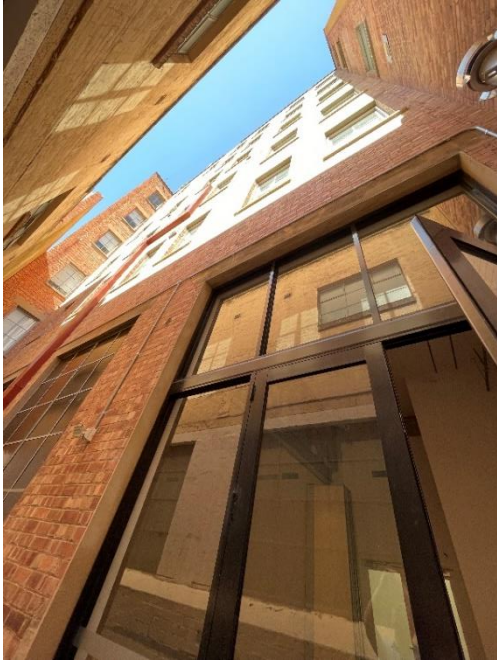
Retrofitted steel doorframe on the east.
