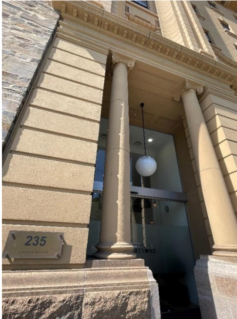
Left front porch on eastern elevation.
