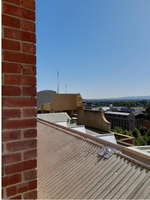
Hipped-roof and rear of the parapet wall.
