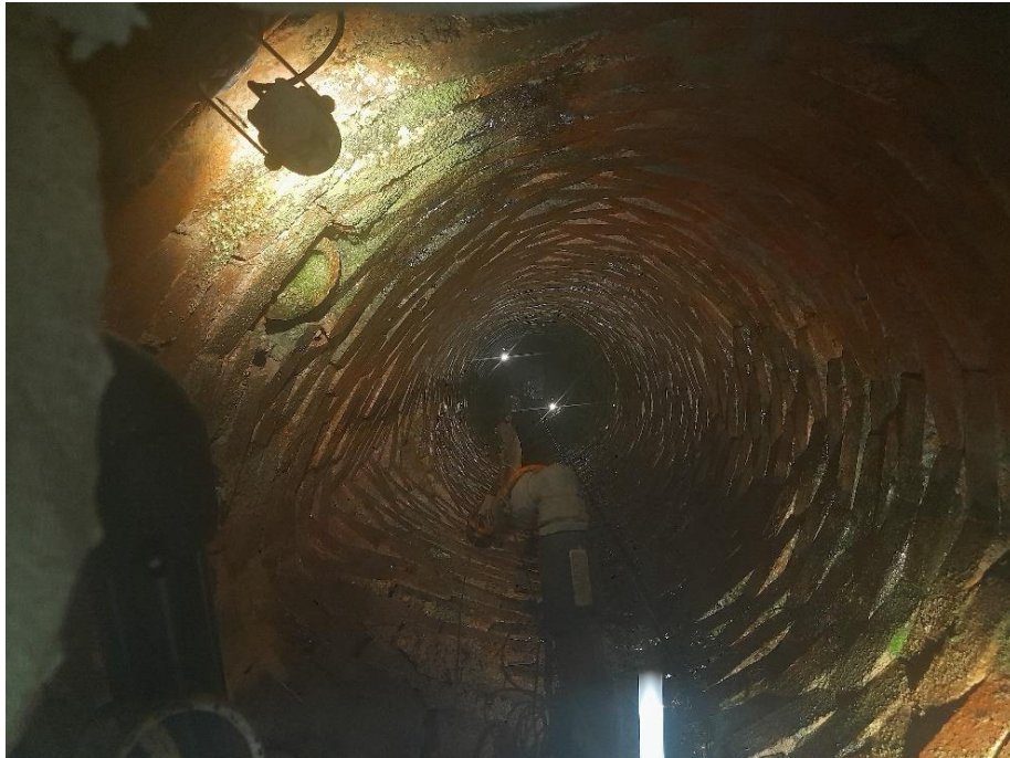
Interior of the sump located in the basement.
