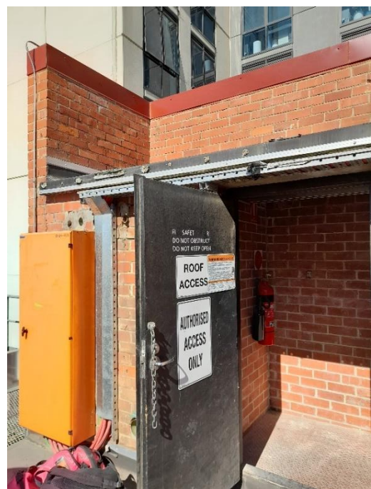
Entrance to roof.
