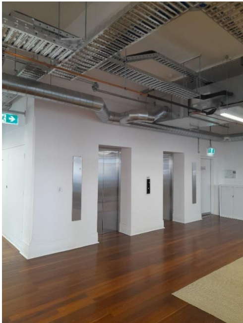
An upper-floor lift lobby.
