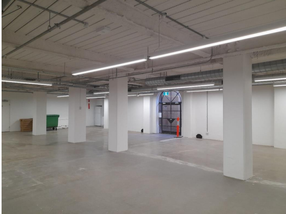
View of the basement entrance showing the steel-framed door facing north.
