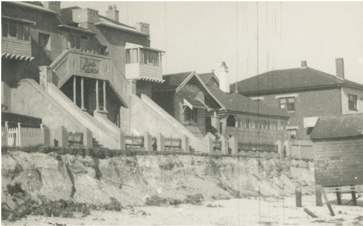
Haigh Mansions (left) and the neighbouring bungalow (right) in 1953, following storm damage to the Henley Beach foreshore, note bathing house on right.
