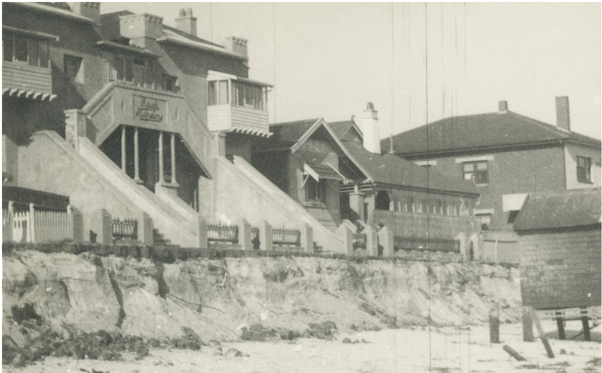
Haigh Mansions (left) and the neighbouring bungalow (right) in 1953, following storm damage to the Henley Beach foreshore, note bathing house on right.
