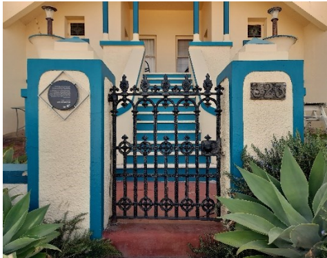
Original cast iron gate
