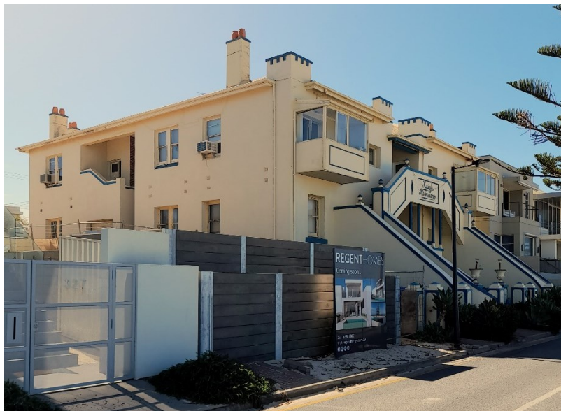
Haigh Mansions, northern and western elevations
