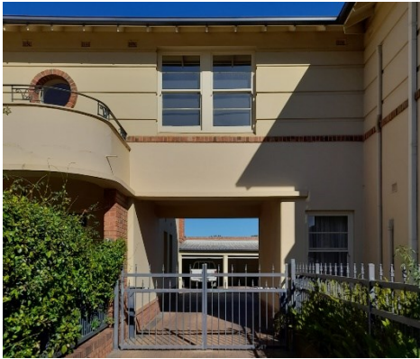
Driveway through main block
