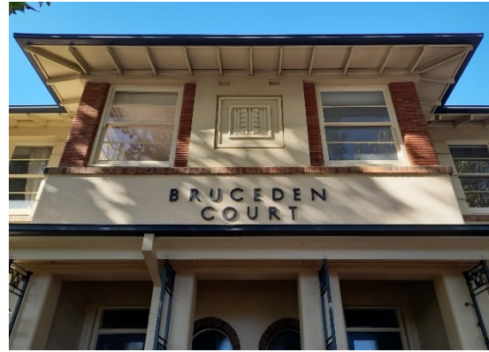
Detail of Cross Road elevation
