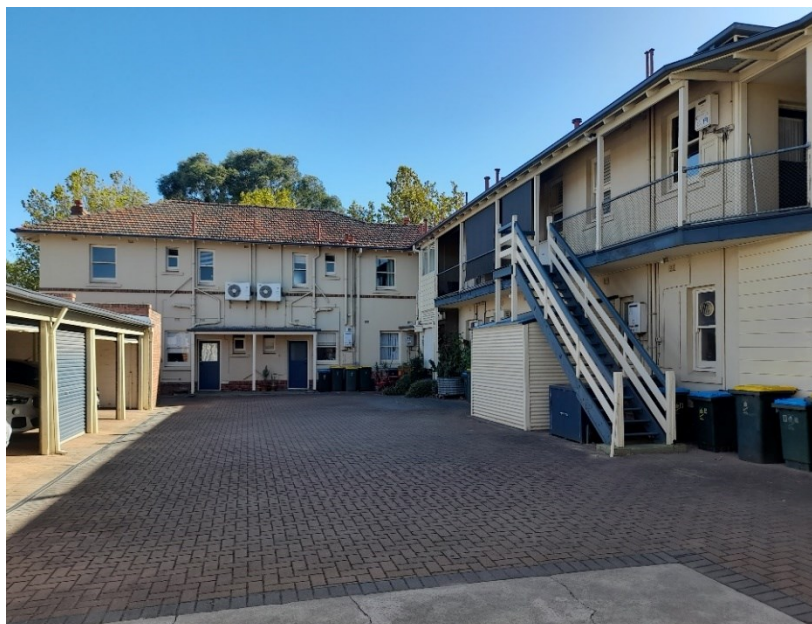
Rear elevations, with garage doors on left
