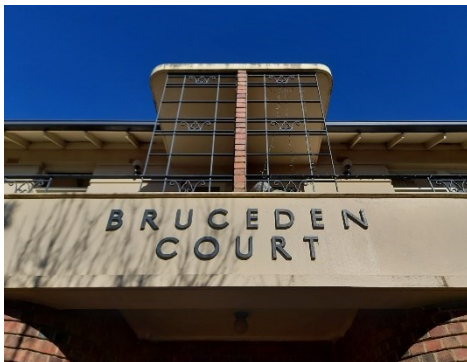
Balcony detail on Deepdene Avenue elevation
