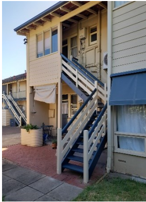
Typical rear staircase structure
