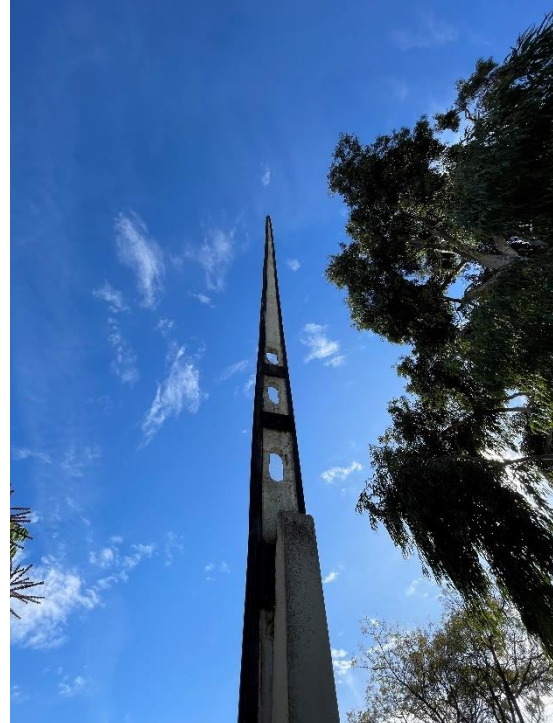
Rear of the 1924 Stobie pole showing tie bolts.
