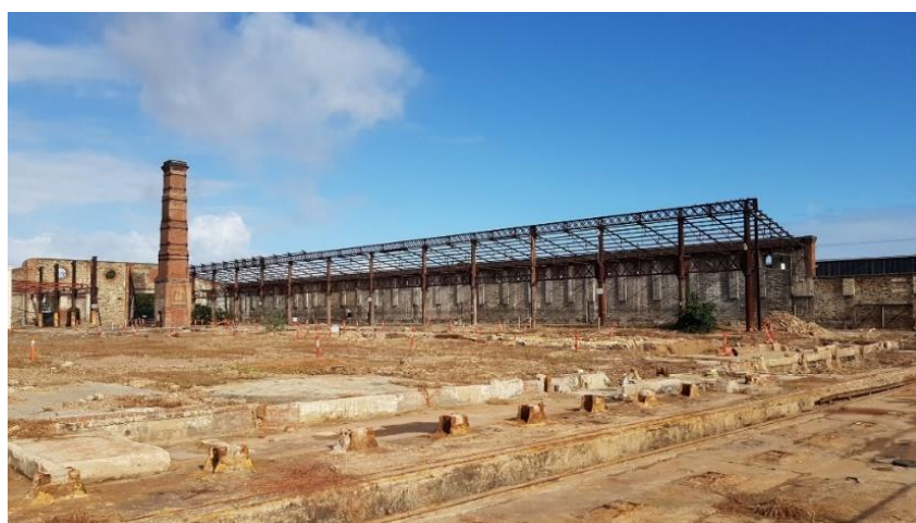
Retort Building and Chimney Stack – Gas Retort (Brompton Gas Works) (SHP 16929).
