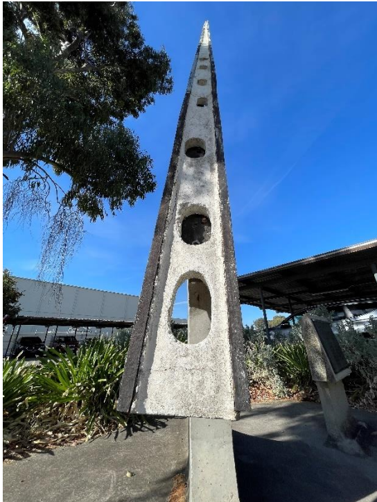
Frontal view of the 1924 Stobie pole showing oval cutouts.
