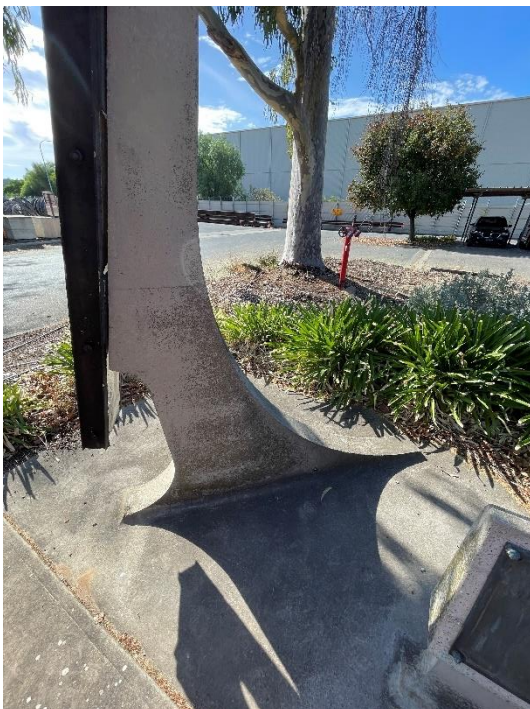
Original concrete base of the 1924 Stobie pole.
