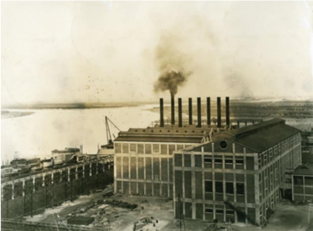
Osborne Power House, c.1927.
