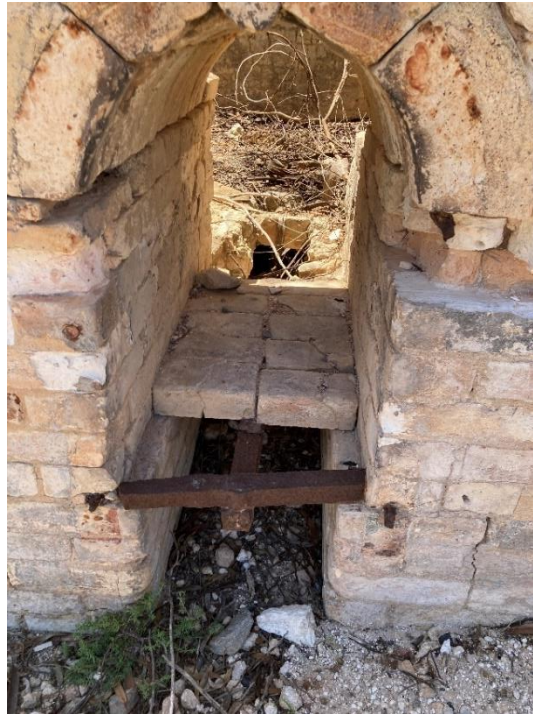
View of the eastern lime kiln firing chamber through the front archway. The elevated chamber is held up by iron bars and bricks, with the ash box below.
