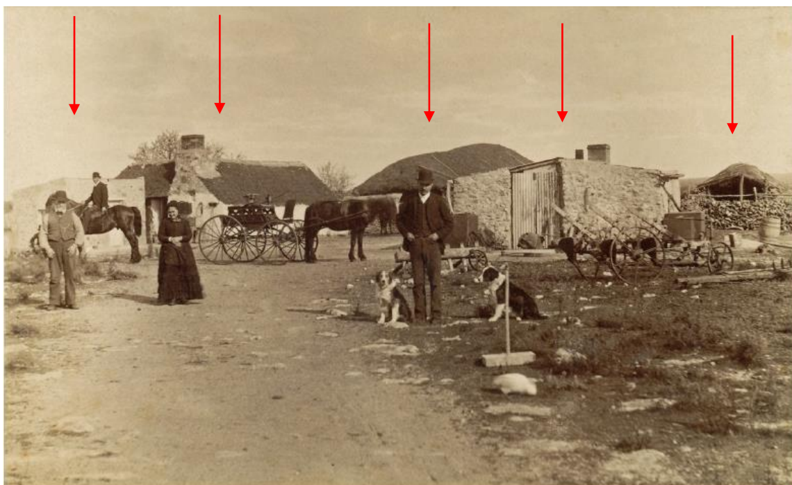
Figure 3. George and Jemima Green at the Trial Farm c.1892. Structures from left to right (indicated by arrows): Limestone room with cellar at rear, earth and stone cottage, wattle and daub cottage, blacksmith's shop, and the mallee root shelter.
