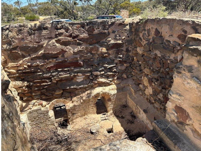
Interior of the eastern lime kiln.
