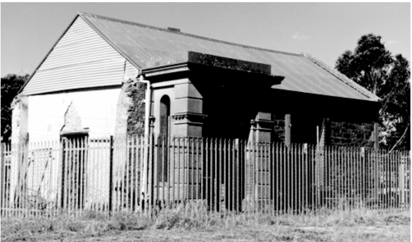
Front view of Lochend, unfortunately the left hand side of the building was demolished during the 1970s, but will be reconstructed in the next stage of redevelopment. The roof covering has been replaced with new galvanised iron.
