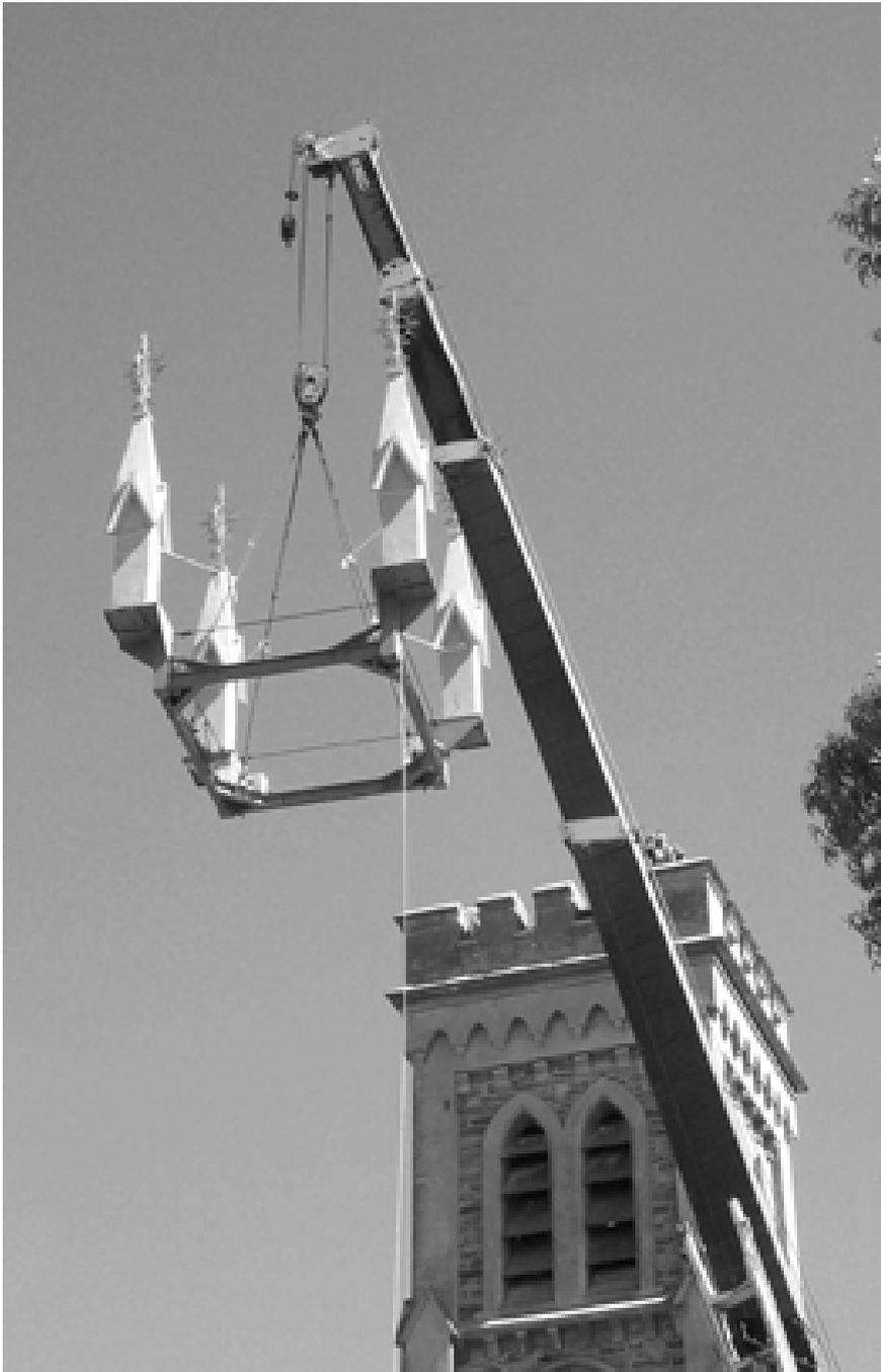
Exposed surfaces of the steel frame were protected against corrosion by grit blasting and applying a single coat of high quality inorganic zinc silicate coating. The frame was fabricated by 'Strath Fabrication and Machining Services'.
