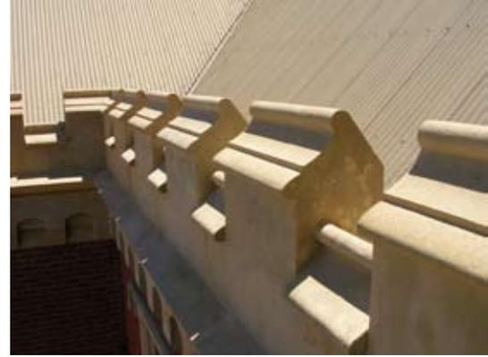
Lime based shelter coat was applied to reconstructed limestone crenulations
