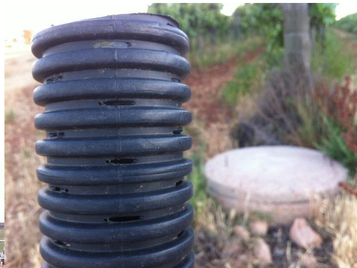
Slotted poly drainage hose installed beneath crop root zone. This collects and runs drainage water into sumps.
