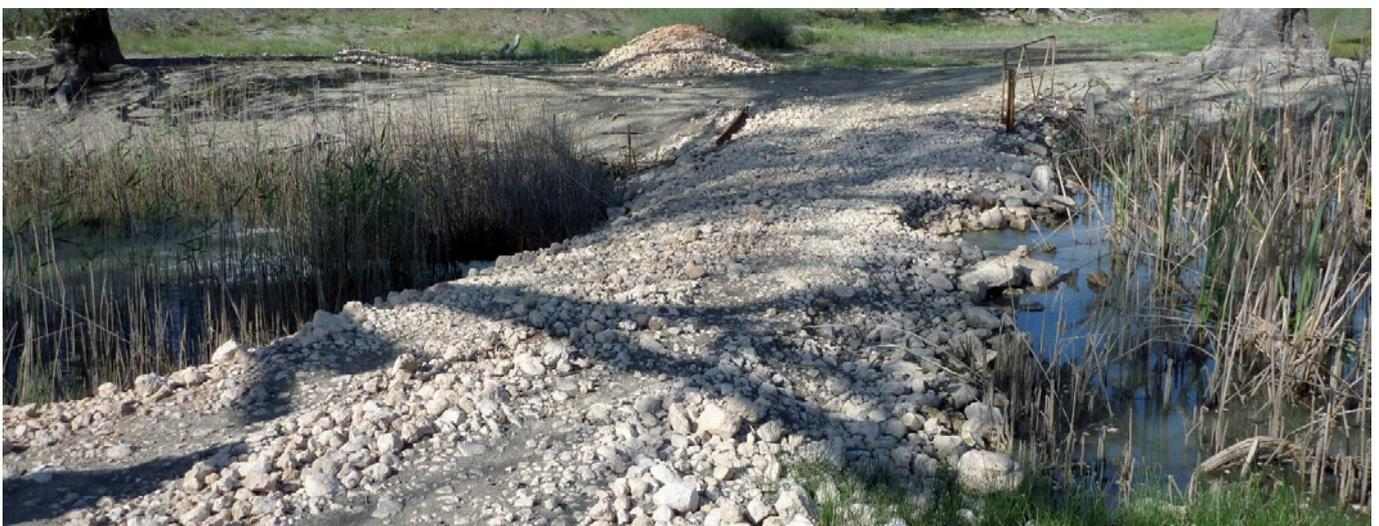
Bank F: one of the crude earthen embankments identified to be upgraded as part of the RRP.
