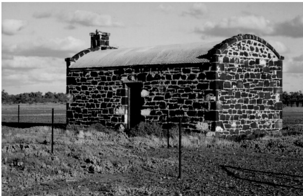
Junction Well Hut
