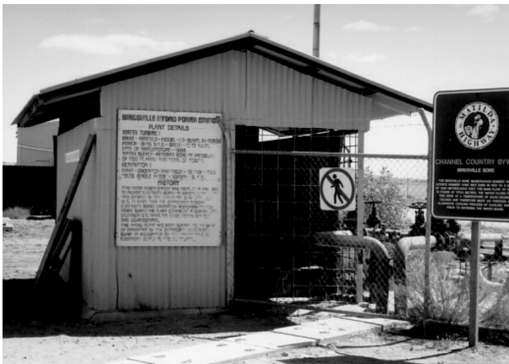
Birdsville Hydro Power Station
