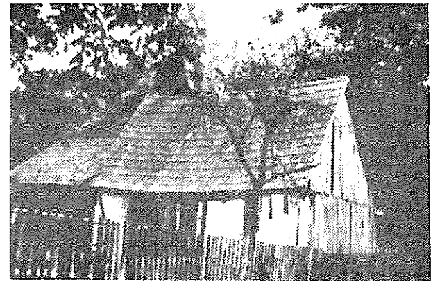
Vertical boarded and shingle roofed barn. Nova Klepsk (Neu Klemzig). Poland 1977. Similar to Schneemilch's barn in Victoria Street.
