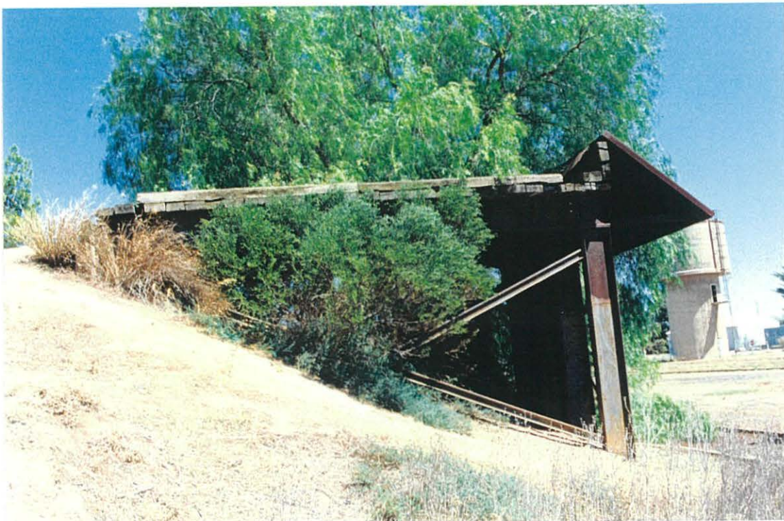
Loading ramp in Kadina rail-yards, 18 January 1995
