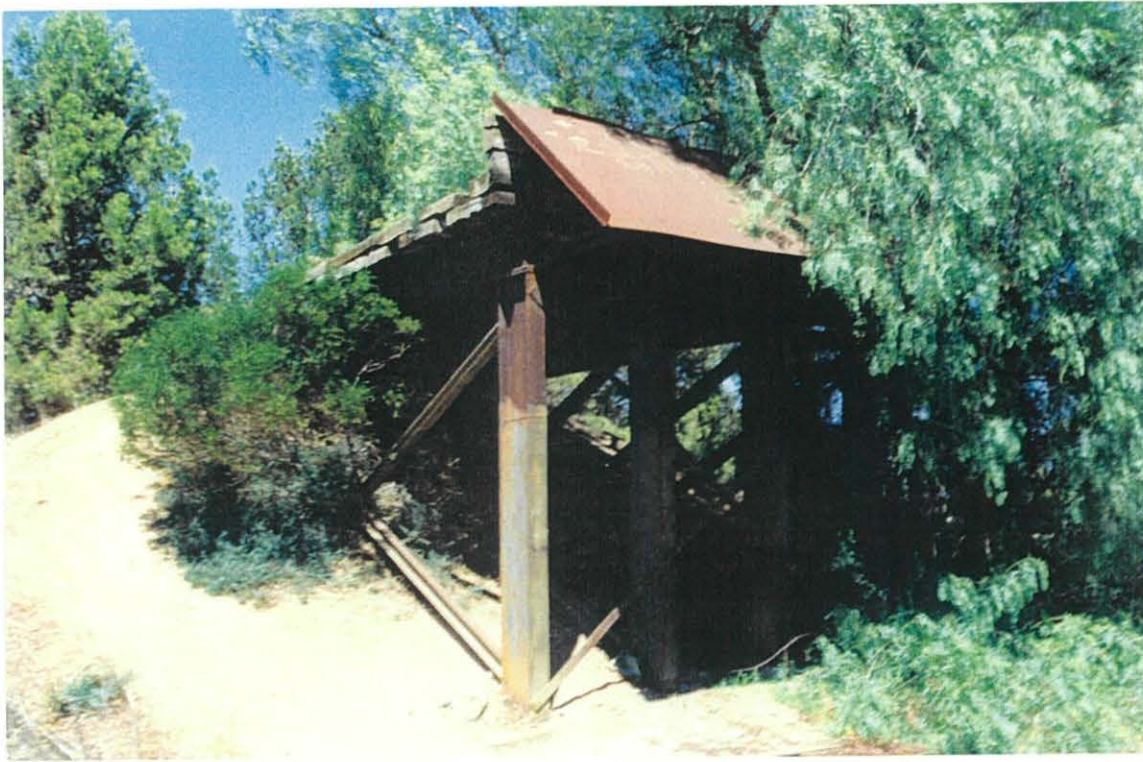
Loading ramp in Kadina rail-yards, 18 January 1995
