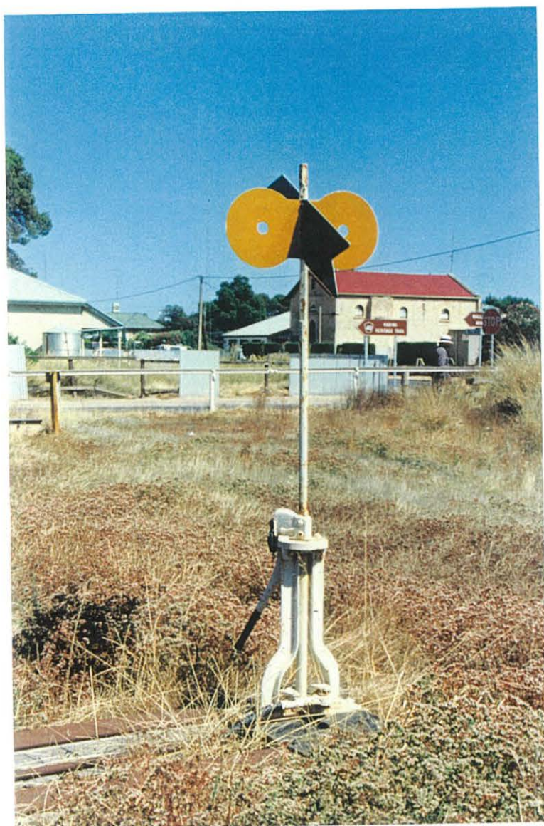
Signal in Kadina rail-yards, 18 January 1995
