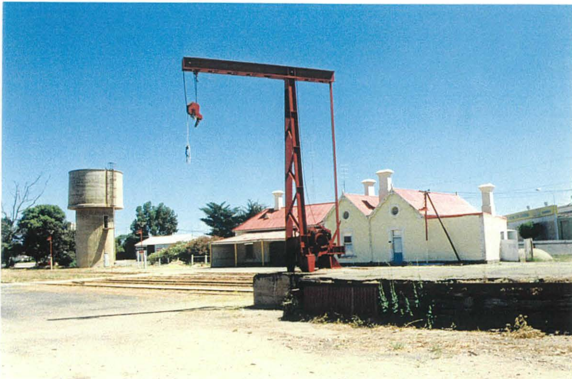
Crane in Kadina rail-yards, 18 January 1995
