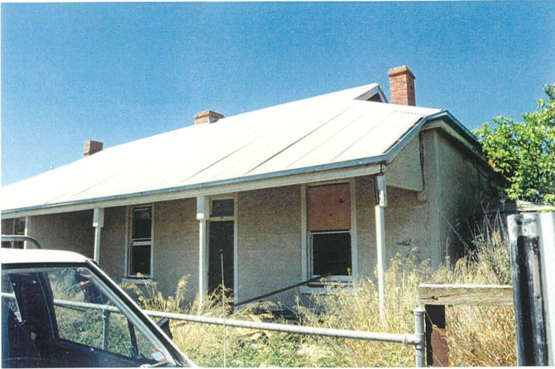
Railway cottage, lot 11, Port Road, 18 January 1995
