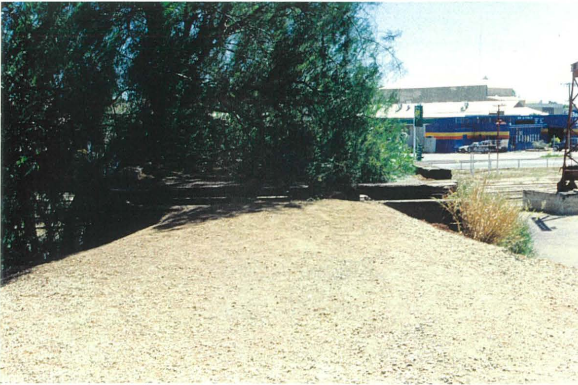
Loading ramp in Kadina rail-yards, 18 January 1995
