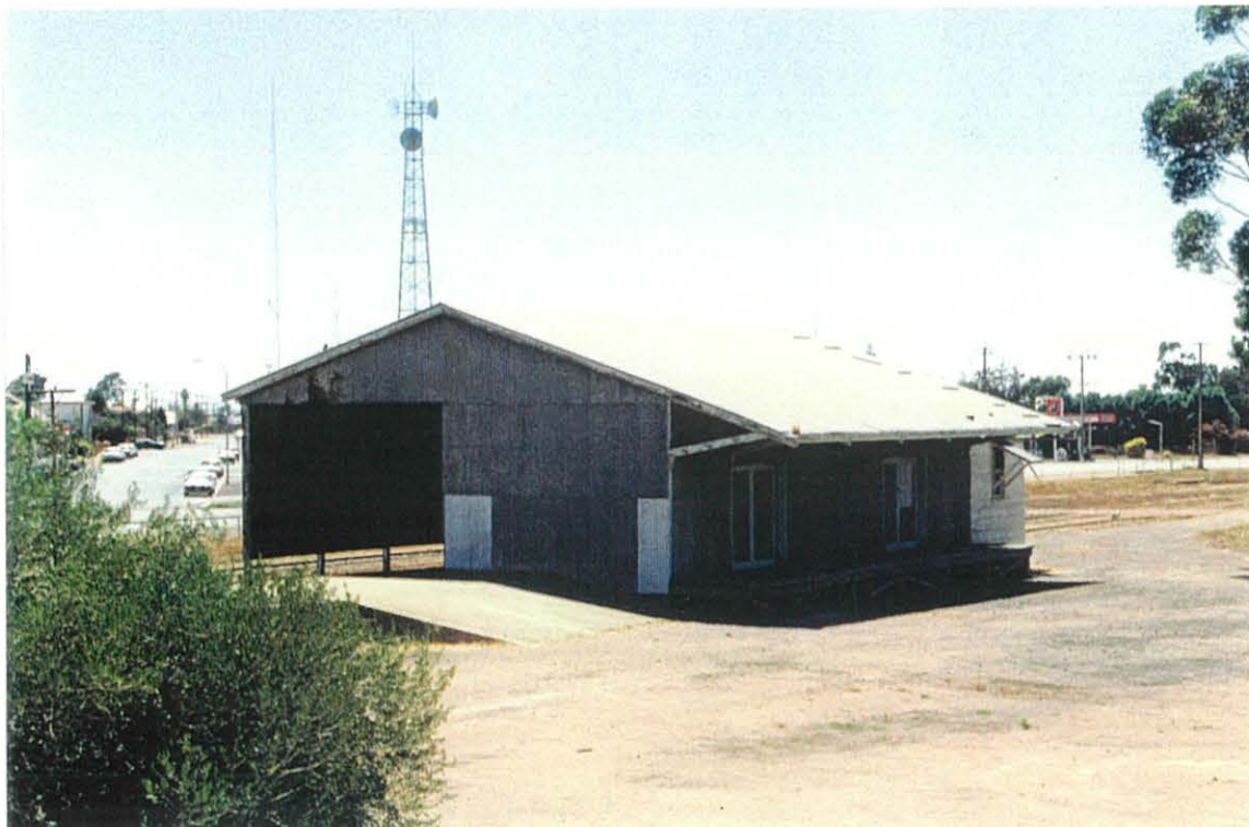
Goods shed (south side) in Kadina rail-yards, 18 January 1995
