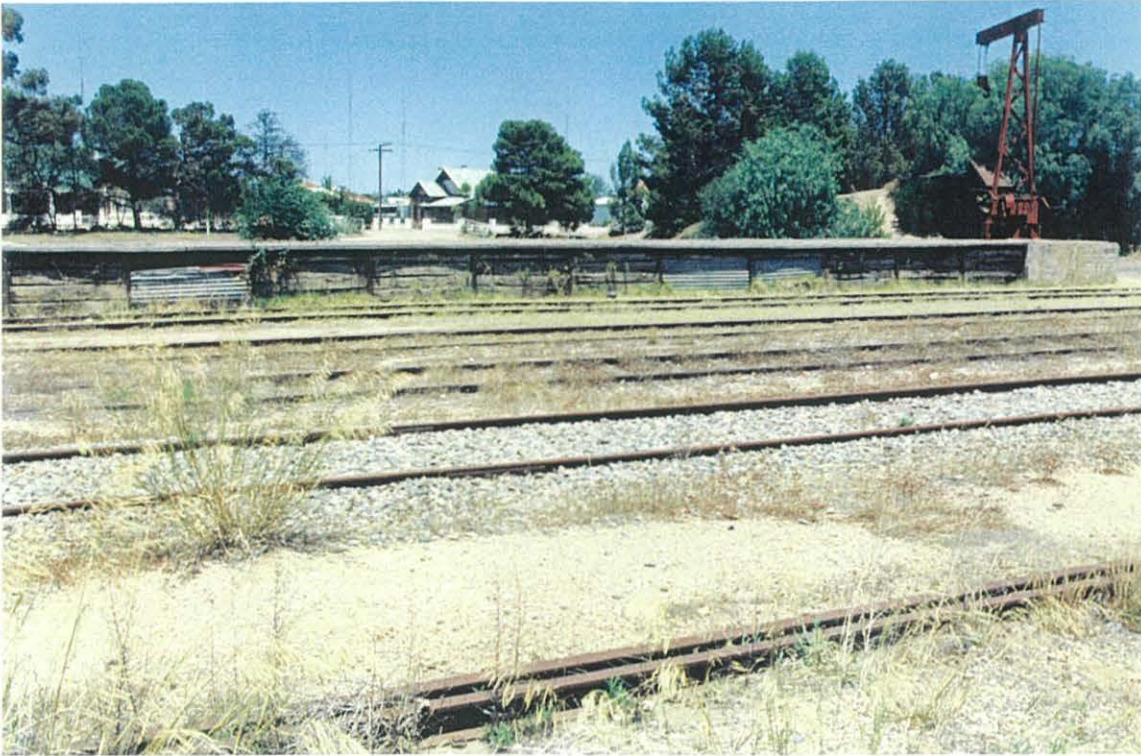
Platform to west of goods shed, Kadina rail-yards, 18 January 1995
