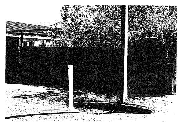
**Description:** Remnant section of the original Victorian bluestone-walled bridge and parapet wall to First Creek. Appears to have been shortened at the southern end.
