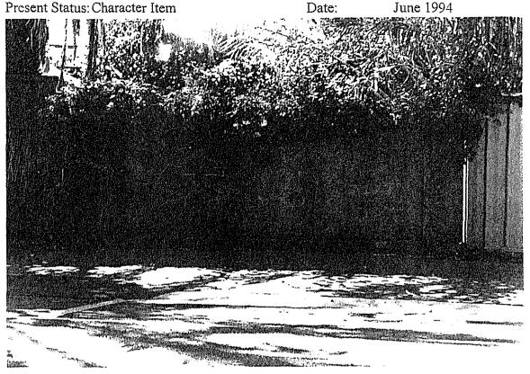
**Description:** A small stone and brick single vault bridge and parapet wall, all of which has been heavily rendered. The piers are at each end of the parapet which has a projecting brick rendered coping and the remains of broken glass.
