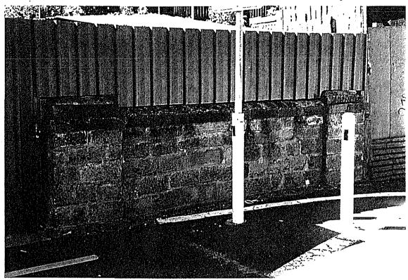
**Description:** This attractive simply built structure is constructed of squared coursed stone with a coarsely punched facing. The bridge consists of a vault with parapet wall. The latter has a panel situated between two piers with simple rectangular copings.
