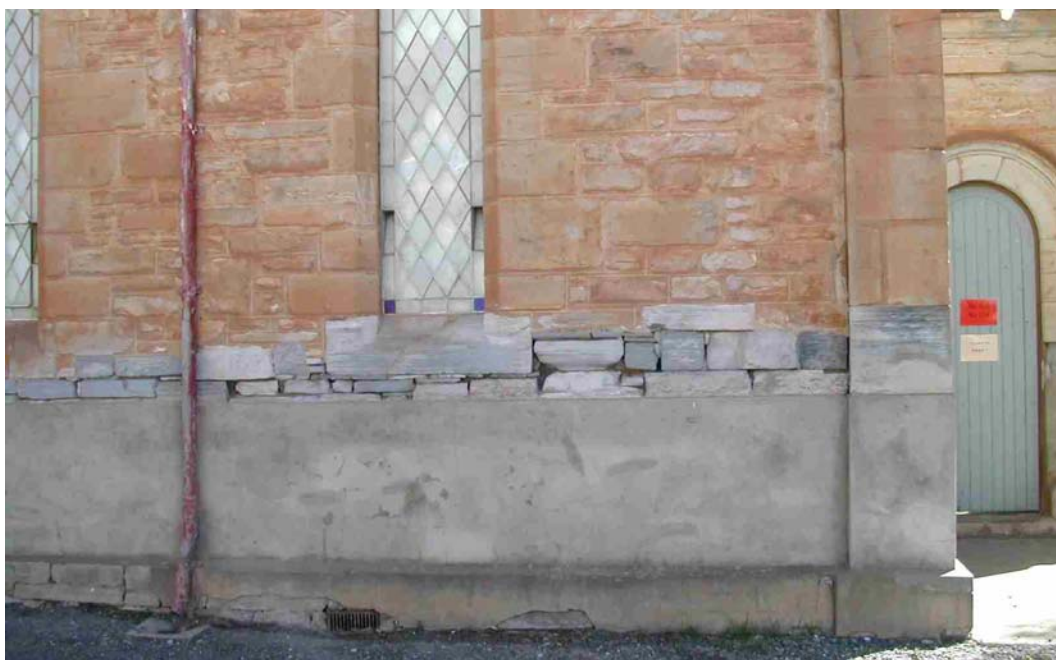
Detail of deteriorating walls
