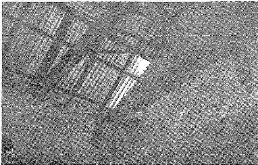
Detail of cob walling to barn, Gumbank. Note the strong horizontal lines which indicate the process of building the walls in layers.
