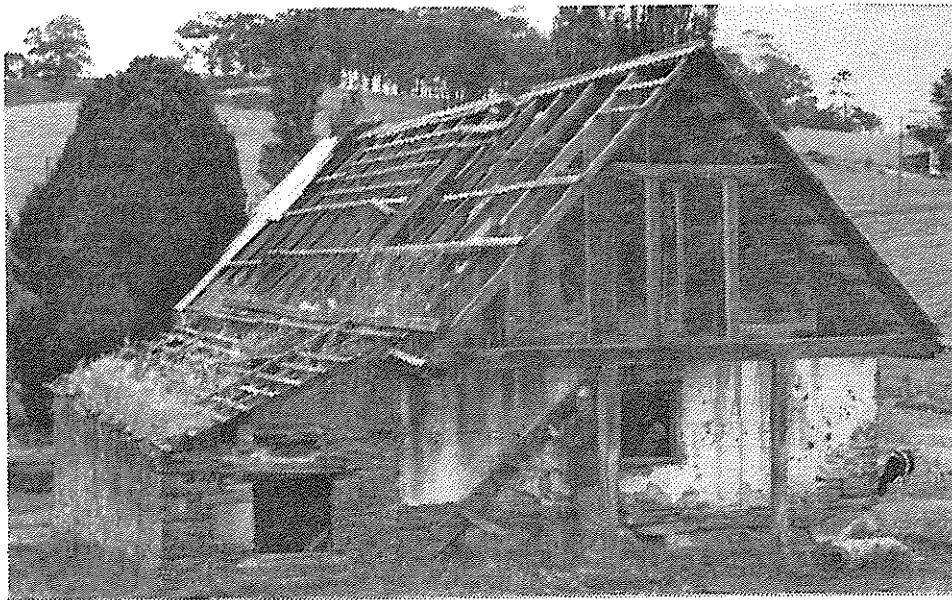
Original house on Section 5103 showing extended gable and collapsed staircase raised in its original position
