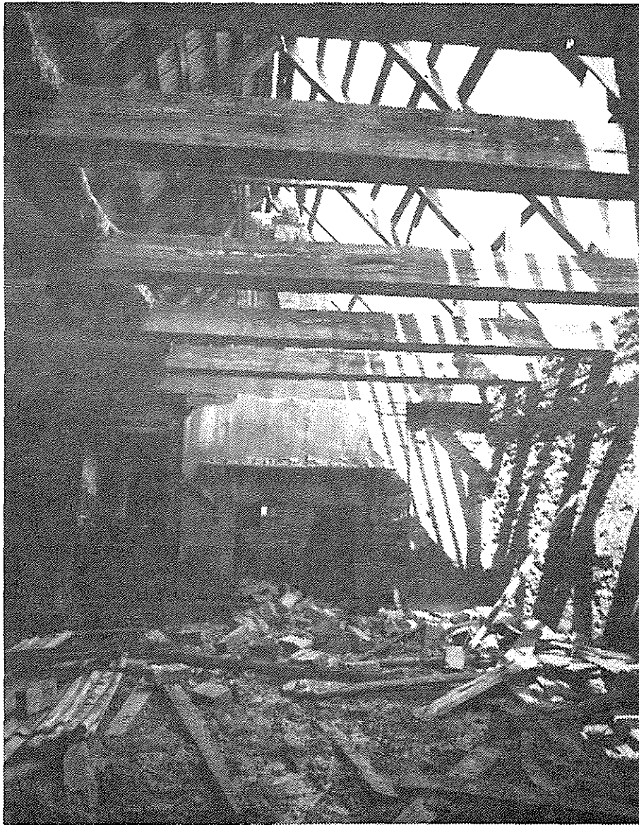
Interior of original house on Section 5103 showing collapsed mud-brick chimney and back-to-back fireplaces
