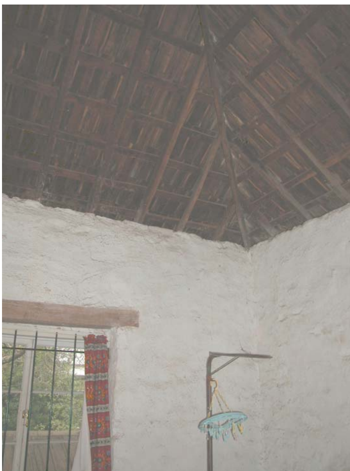
Interior of fr Johnson's mill showing timber lintels and shingles, 2004
