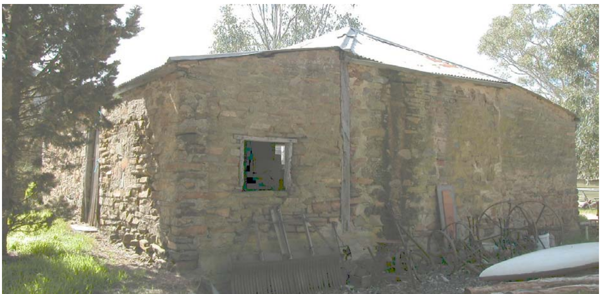
Original cottage at Mount Farm – note timber posts within walls, 2004
