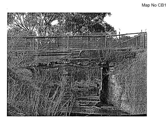
A former road bridge with a single central stone pier, stone buttressing and local, rough-sawn timber log construction.
