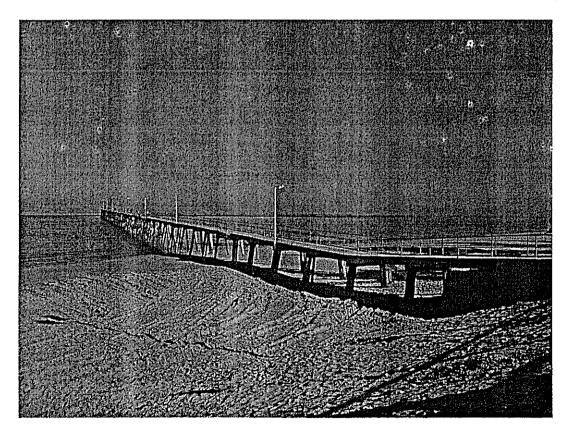
The jetty is 1080 feet long and 8 feet wide, and is constructed of ...
