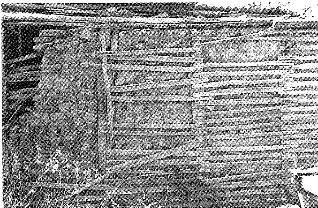
Lath and plaster walling showing stone infill
