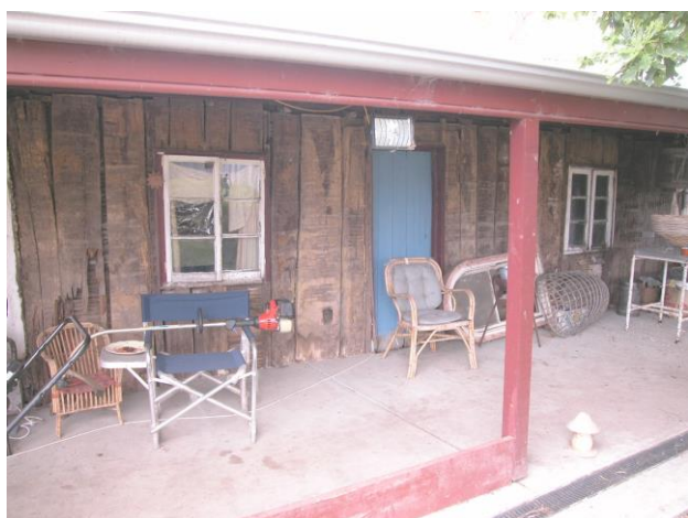
Timber-slab wall, 2 Rohrlach Street
