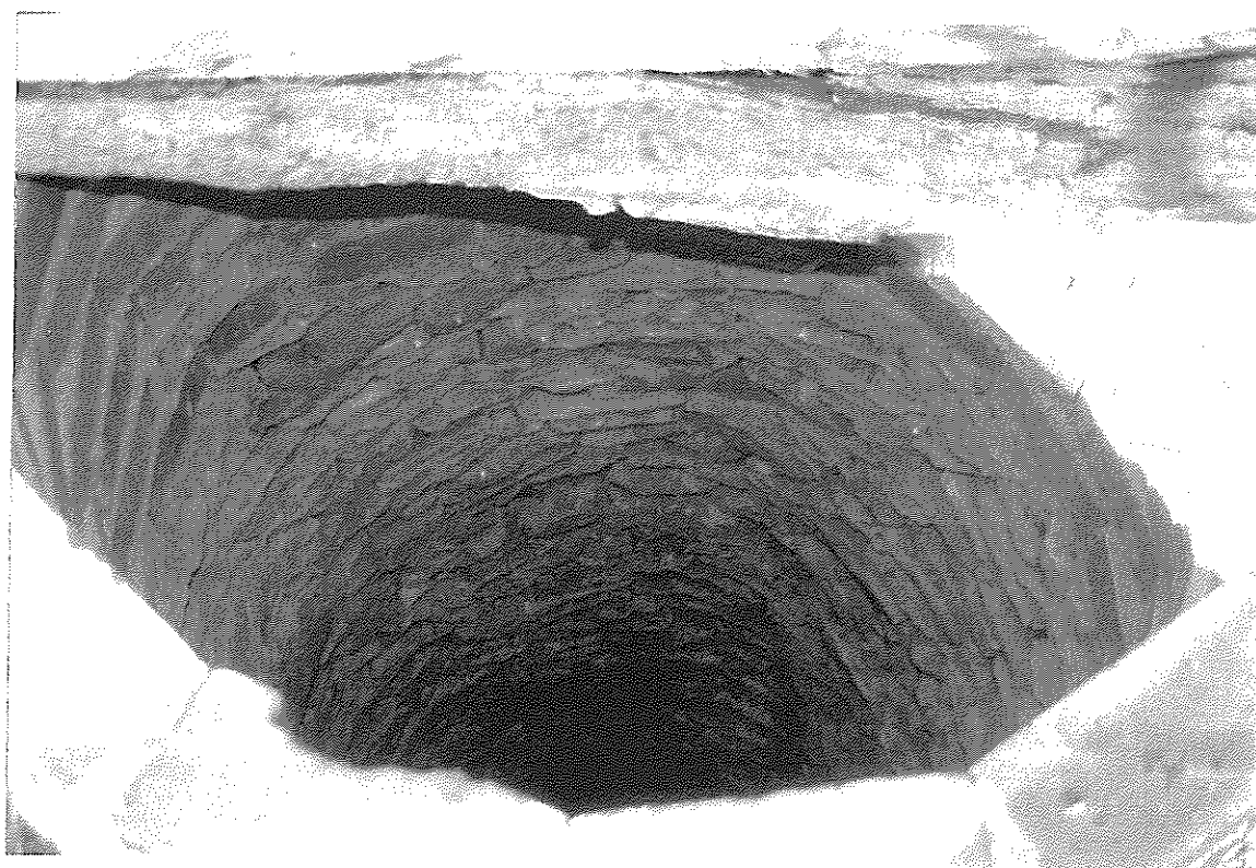
Note: brick edge and stone lining
