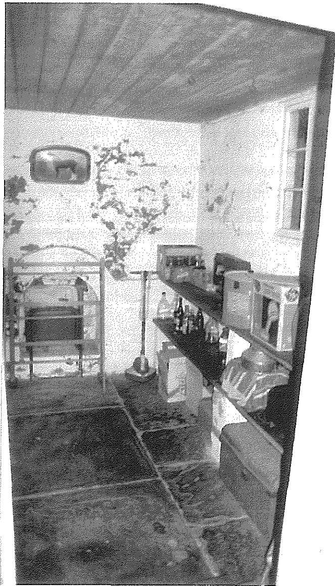
Interior of cellar - note slate flags and shelving
