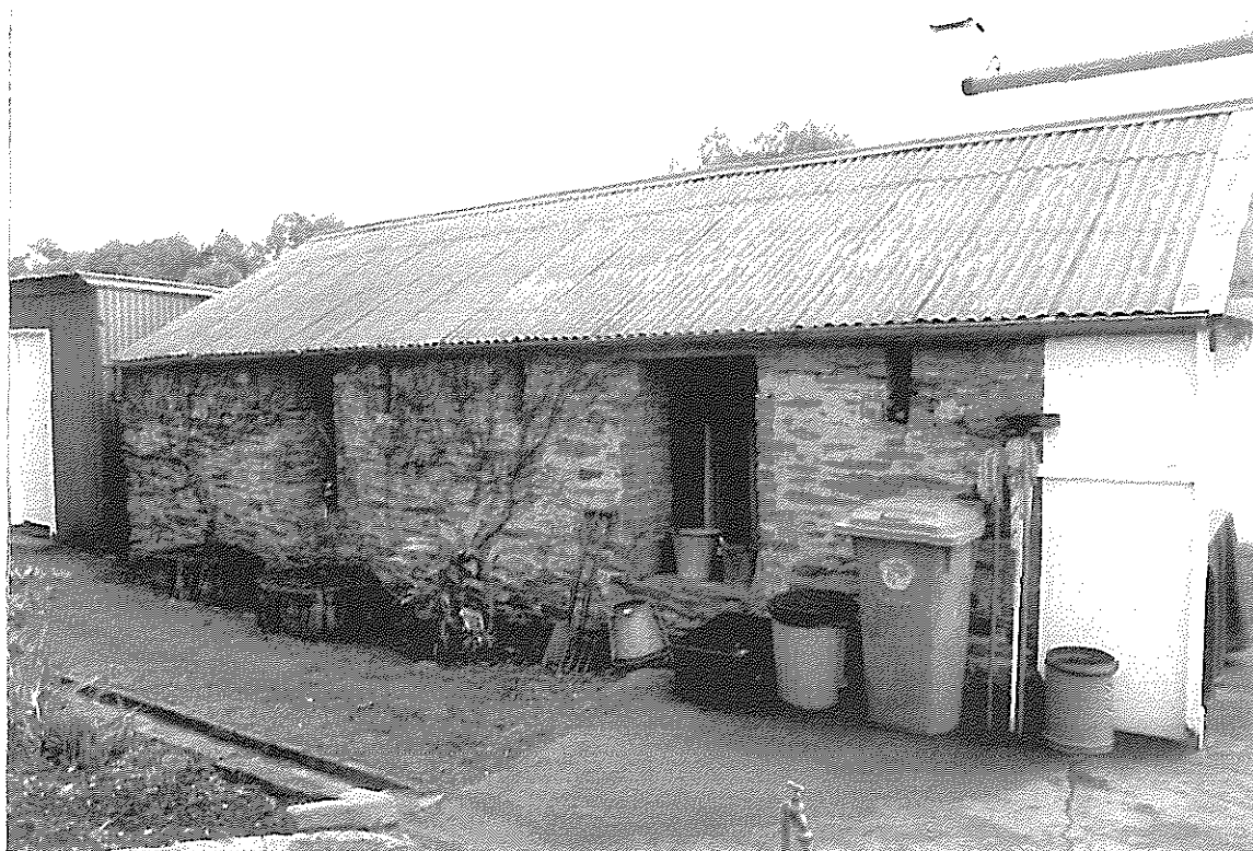
Stone side walls of external cellar
