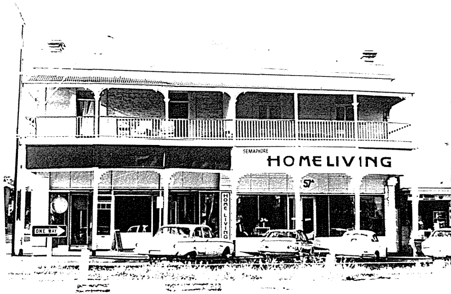
57-57A Semaphore Road. 1979 Photograph - prior to removal of railway and rebuilding of verandah.
