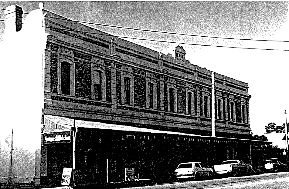
Shops 11-15 Jetty Road
