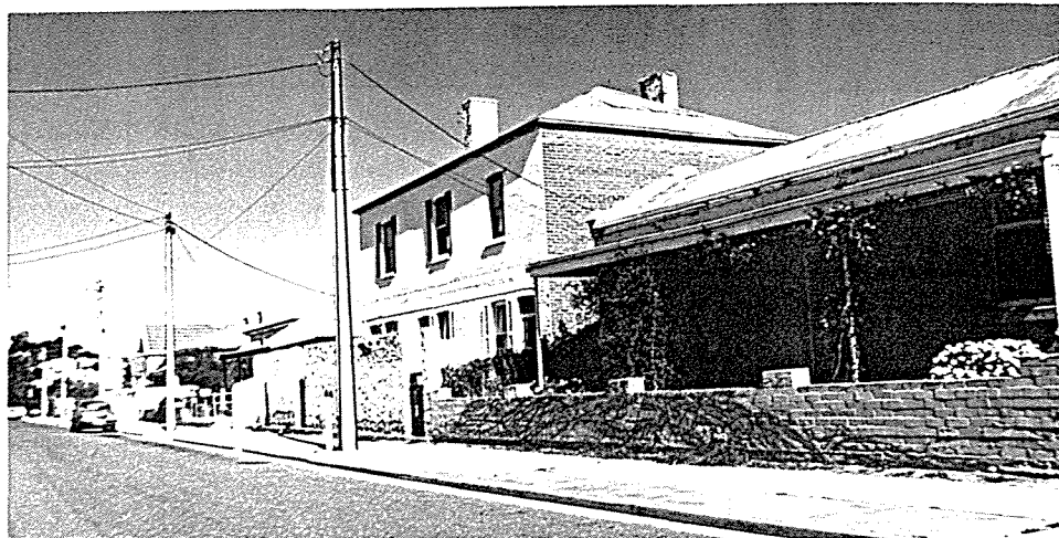
Montpelier Street, West side
