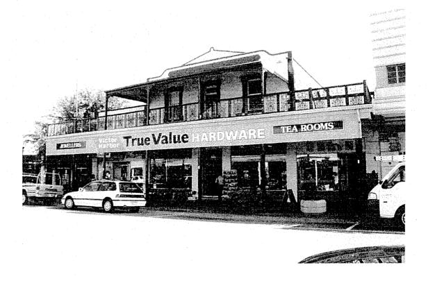
A double-storey shop constructed of local limestone with a wide verandah/balcony, and ornamental pediment above, behind which is a pitched corrugated galvanised iron roof. A central doorway with fanlight above opens on to the balcony with timber framed double hung sash windows each side of the door. The ground level shop fronts appear to be original, metal framed, with (re)tiled stallboards. The wide balcony balustrading is not original.
