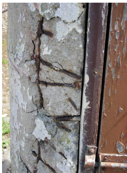
Views of corroding metal reinforcing
