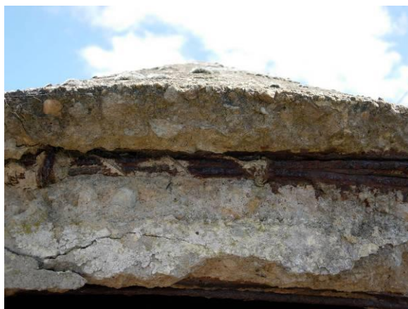
Views of corroding metal reinforcing
